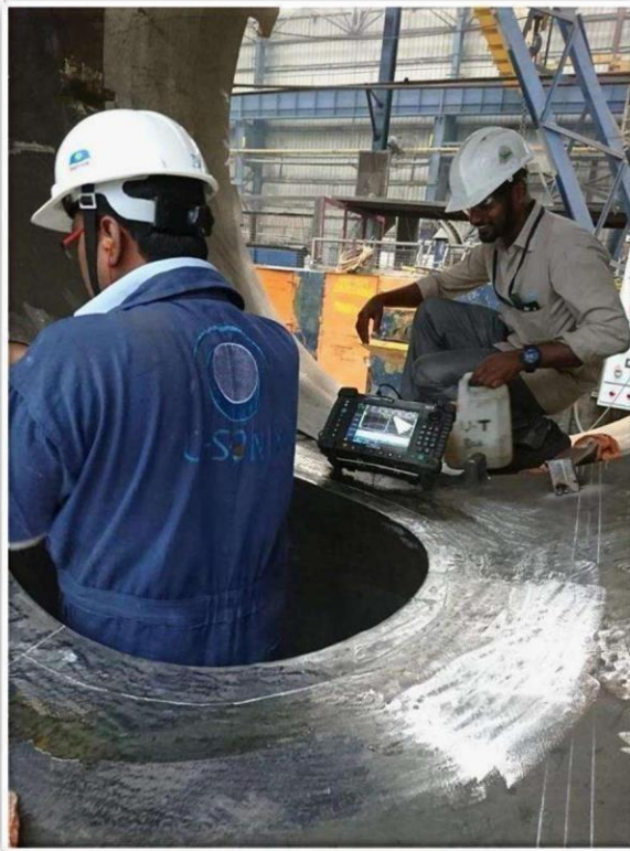
PAUT Inspection of Shell Nozzle at ISGEC Yamuna Nagar
