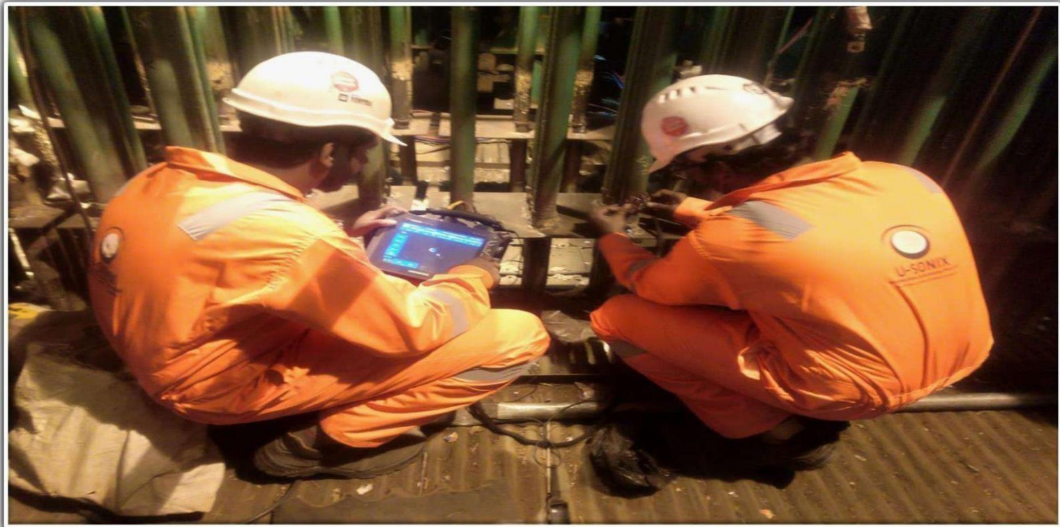
PAUT Inspection of Boiler Tubes at NTPC Barh
