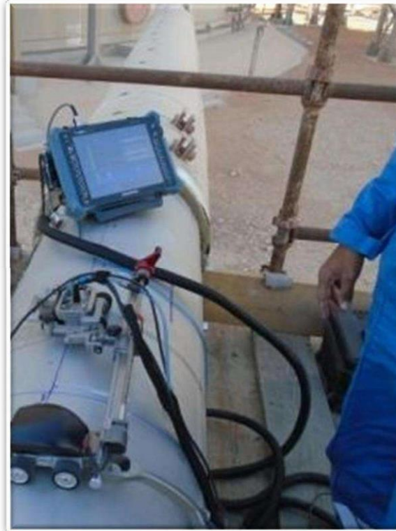
Hydroform Corrosion Mapping - Velosi Oman
