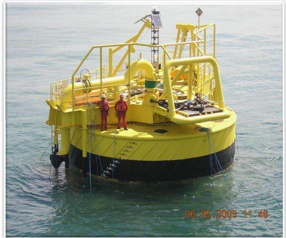
SBM Installation Inspection - Ghana
